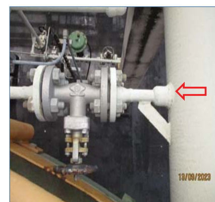
Picture 6 Small-bore and Gusset plate
