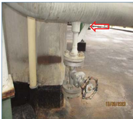
Picture 11 Small-bore and Gusset plate
